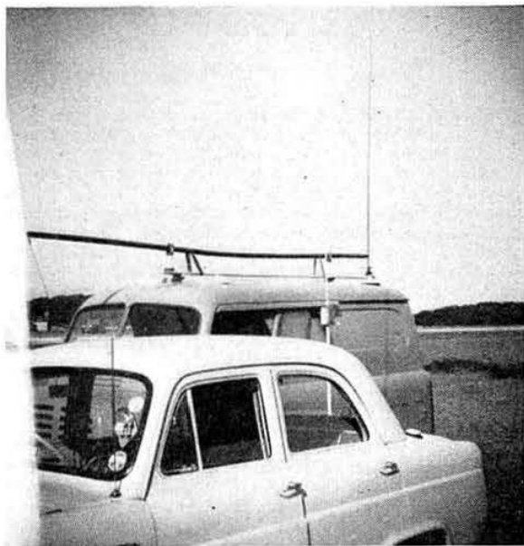
The longest loading coil of all, belonging to G3ERN/M, was installed on top of a Bedford van. The whip can be seen at the rear of the roof. By comparison, G3CIM's loaded whip mounted on the Ford Prefect (foreground) was very modest indeed. (Photo by G2AHL)
